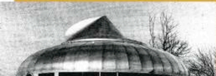
dell'acqua / Buckminster Fuller's Wichita Dymaxion House was one of the first designs to optimise and standardise how detached houses were made. The frame hangs from a central support which also carries the electrical
